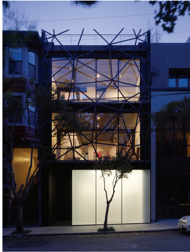
Figure 1. Delaunay Lattice , San Francisco, 2009. Facade lattice generated by self-avoiding agents and triangulation algorithm.
